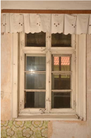
1.02, Wand a, Fenster
